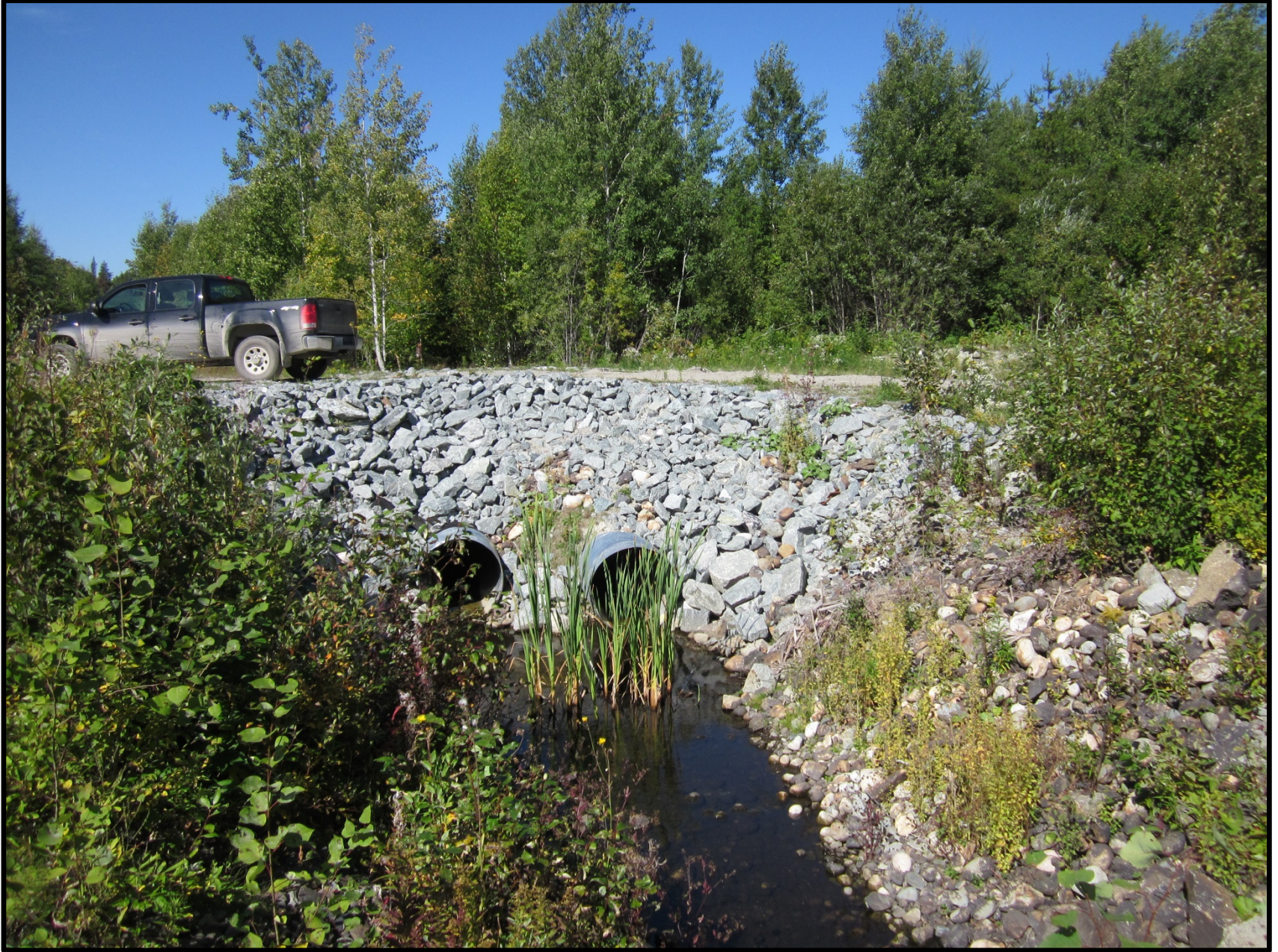
Photograph 3: Dam 4B, final effluent area
