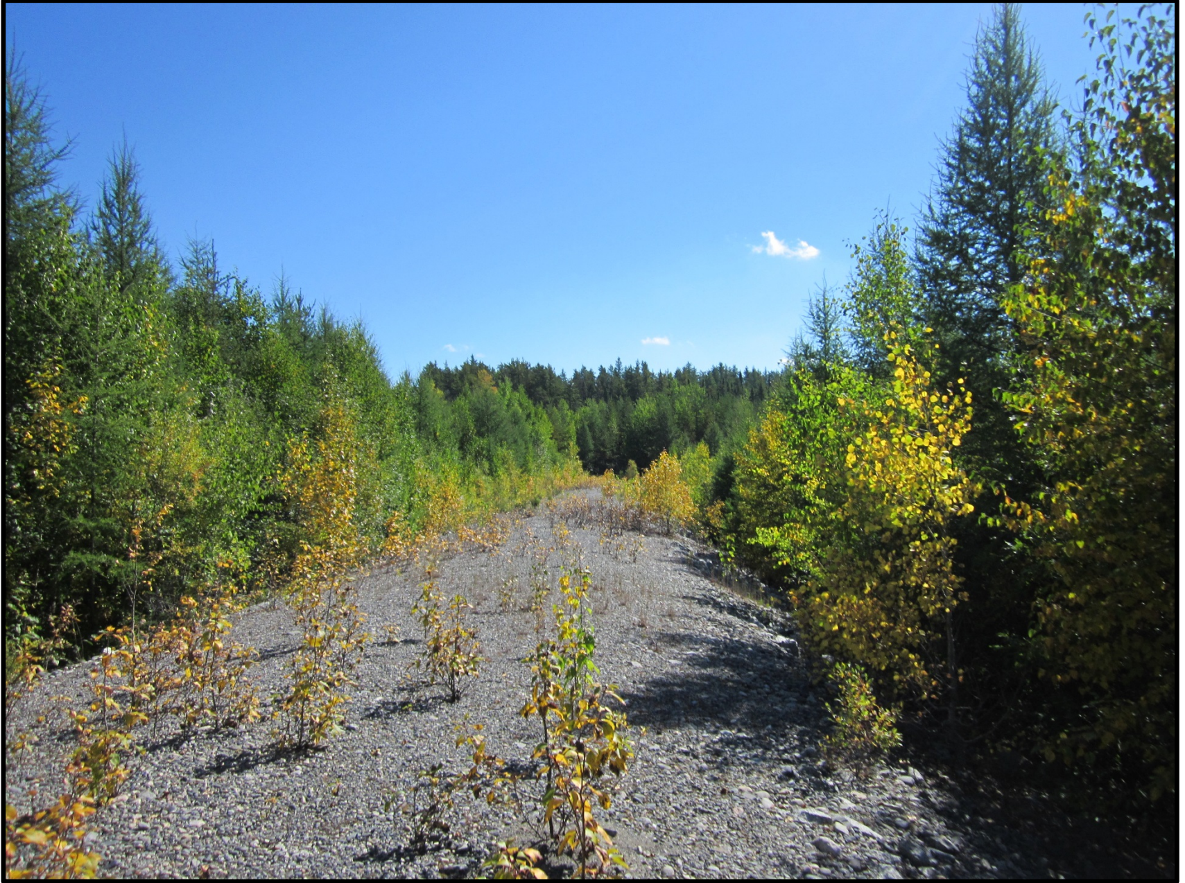
Photograph 1: Louvicourt Mine, Dam 4A
