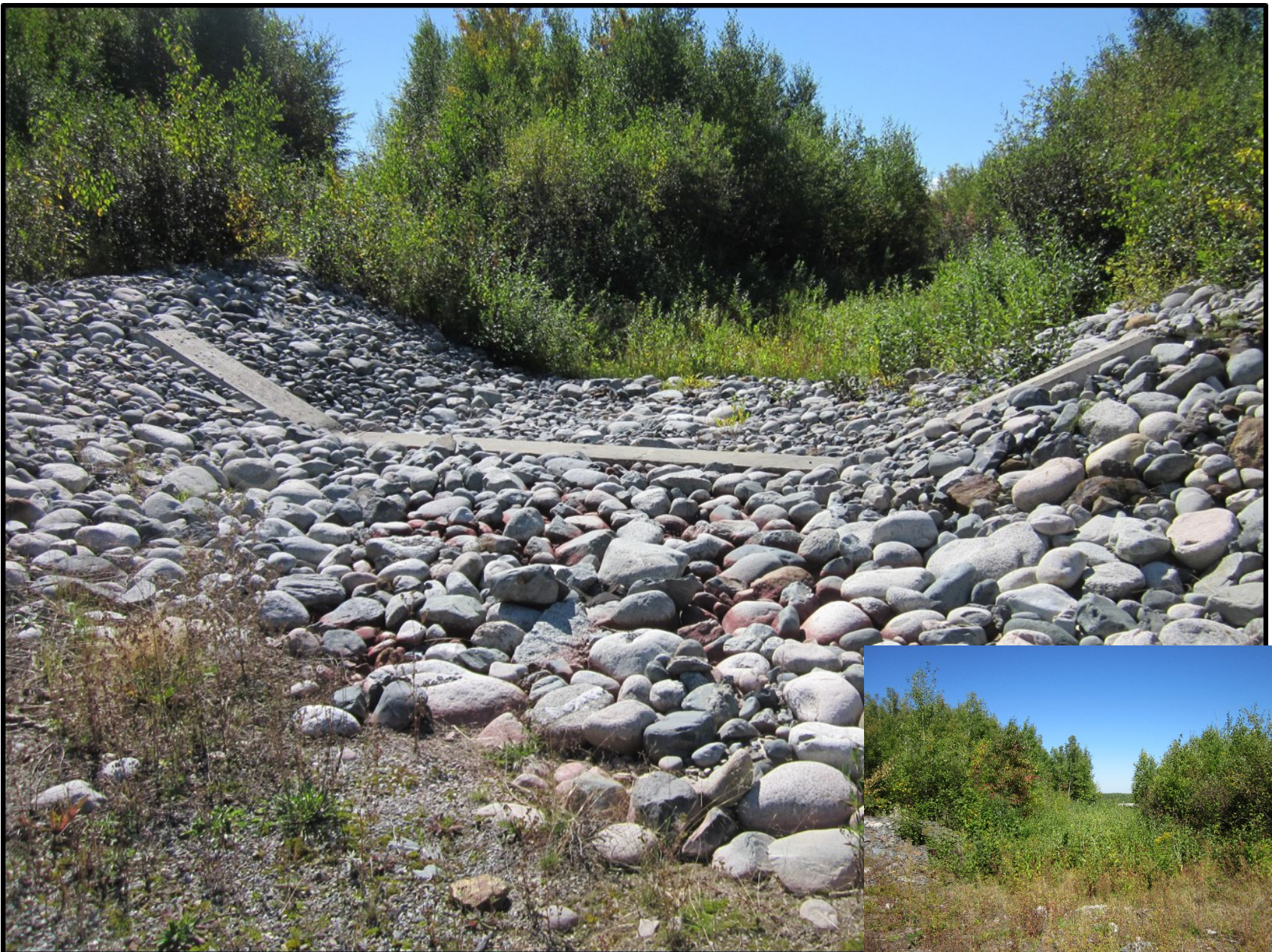
Photograph 7: Dam 1E, emergency spillway
